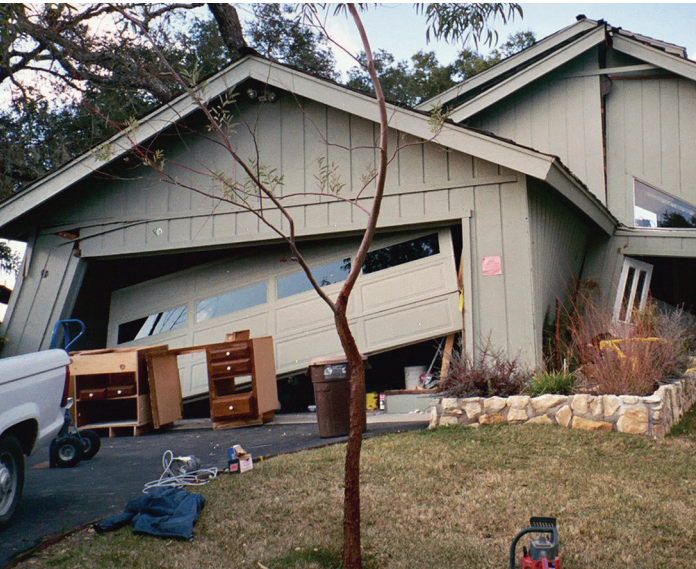
(ABOVE) ATASCADERO, CA JANUARY 25, 2004 -- THIS HOME SLID TWO FEET OFF ITS FOUNDATION DUE TO THE 6.5 SAN SIMEON EARTHQUAKE. PHOTO BY DANE GOLDEN / FEMA NEWS PHOTO
